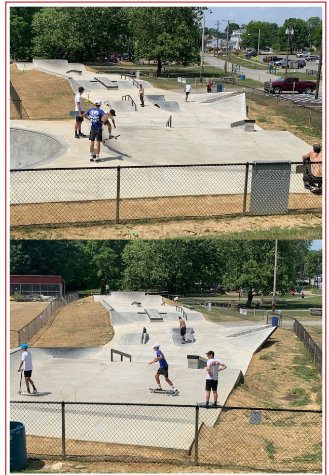
After years of planning, the Zelienople Memorial Skate Park is finally complete.
